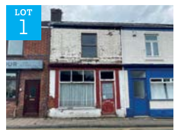
44 Farnworth Street, Widnes, Cheshire WA8 9LH
