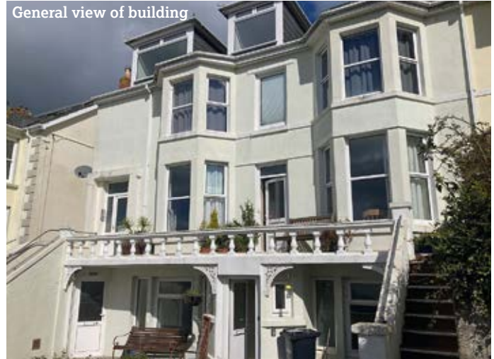
General view of building
